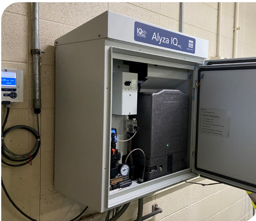
Alyza IQ PO4 analyzer installed at the effluent of Oconomowoc WWTF, providing feedback for automatic ferric dosing control.
